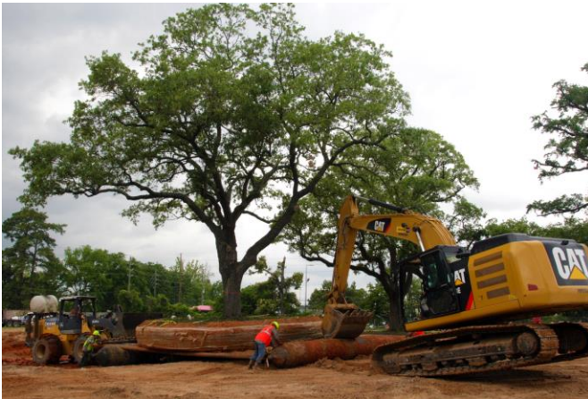
PHOTO CAPTION: The Environmental Design & Davey team relocates a 60-foot-tall, 35" diameter 100-year-old live oak tree using what's known as a roundball transplant technique.
