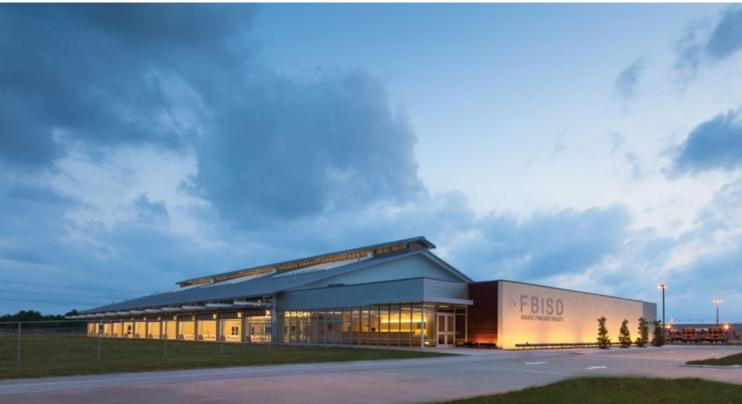
In the spirit of innovation, 23 overhead doors double as shading devices when open on the east and west sides to direct the prevailing seasonal winds.
